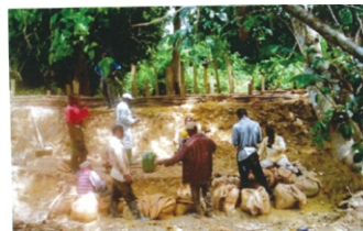
Photo. 3-23. Excavation of river bottom and jute bags
