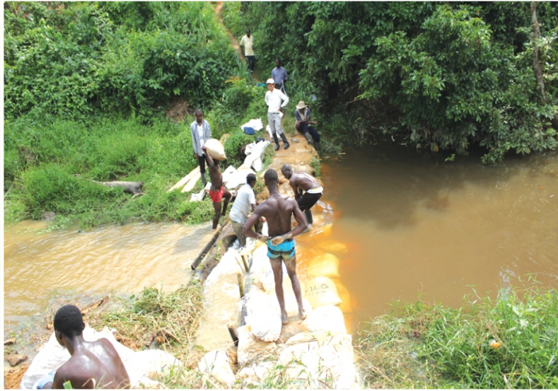
Sand bag and Wooden Weir, construction through farmers' self-support management in Ghana (1999)
